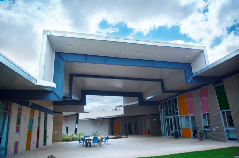
School of Creative Arts Building - Townsville
